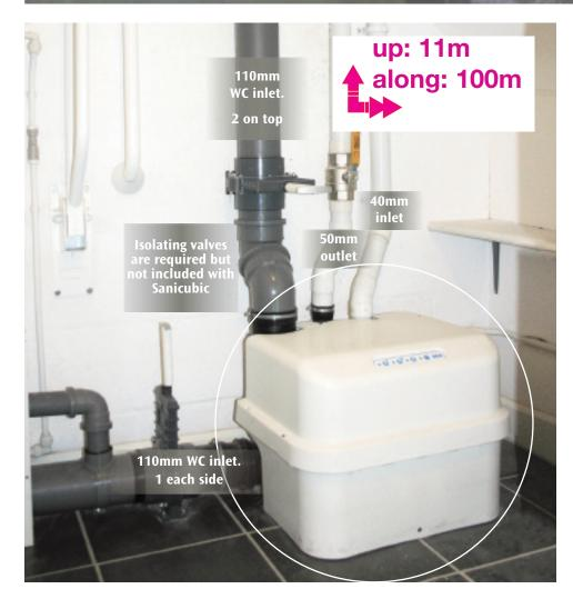
Sanicubic unit has been installed in the basement of the cottage to pump waste and water to the mains, which is situated some distance away.
