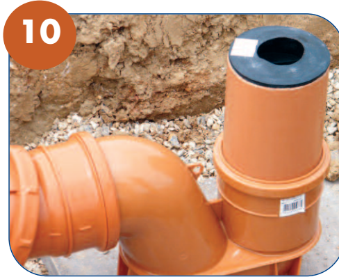
✓ Rainwater downpipes connect to the system via a Universal Rainwater Adaptor.
