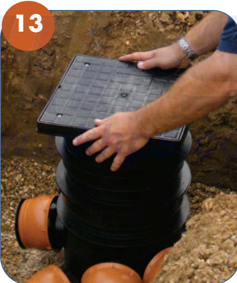
✓ Mini Access Chambers can be added up to a maximum height of 600mm. ✓ Large Inspection Chambers can be up to 1.2m in height with the standard 450mm frame and lid. ✓ Up to 3m using a 350mm reduced access frame and lid.
