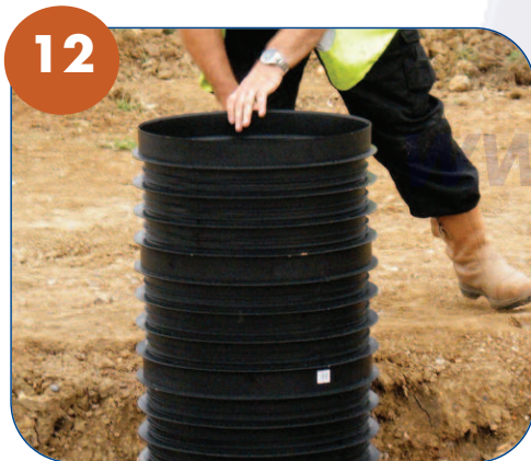
✓ To complete the installation of Inspection Chambers, add risers to the required depth.
